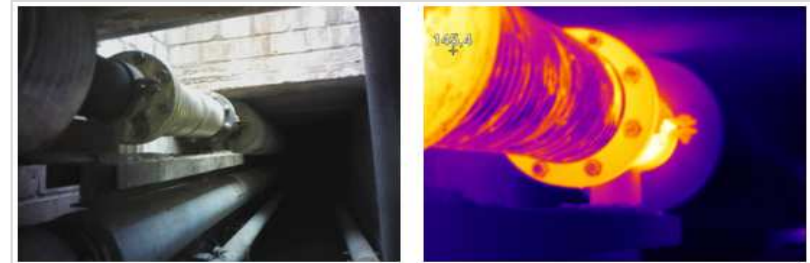
Exposed expansion joints
